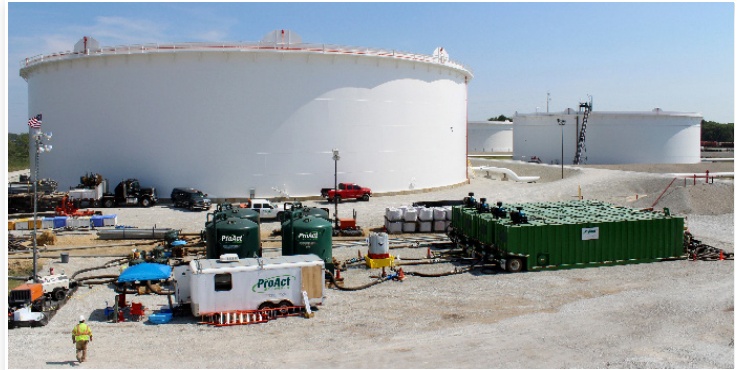
2000 gallon per minute water treatment system
